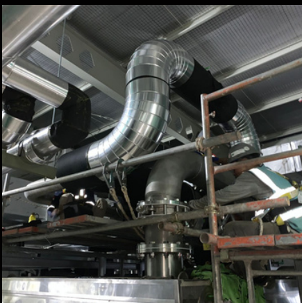
Insulasi Chiler Pipe
