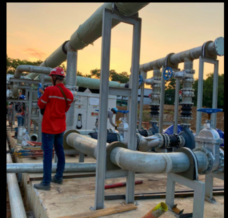
Instalasi Pipa Chiller GLV
