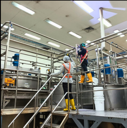
Instalasi Pipa Sanitary
