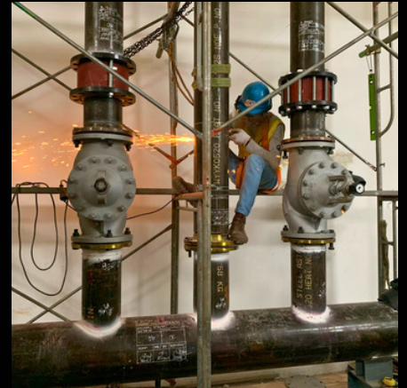
Instalasi Pipa Steam
