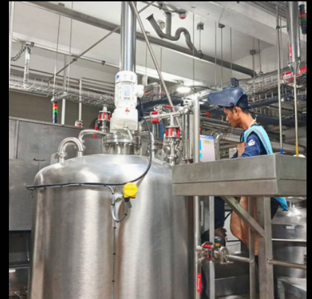
Instalasi Pipa Sanitary
